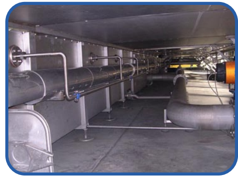
CIP Pipe work
